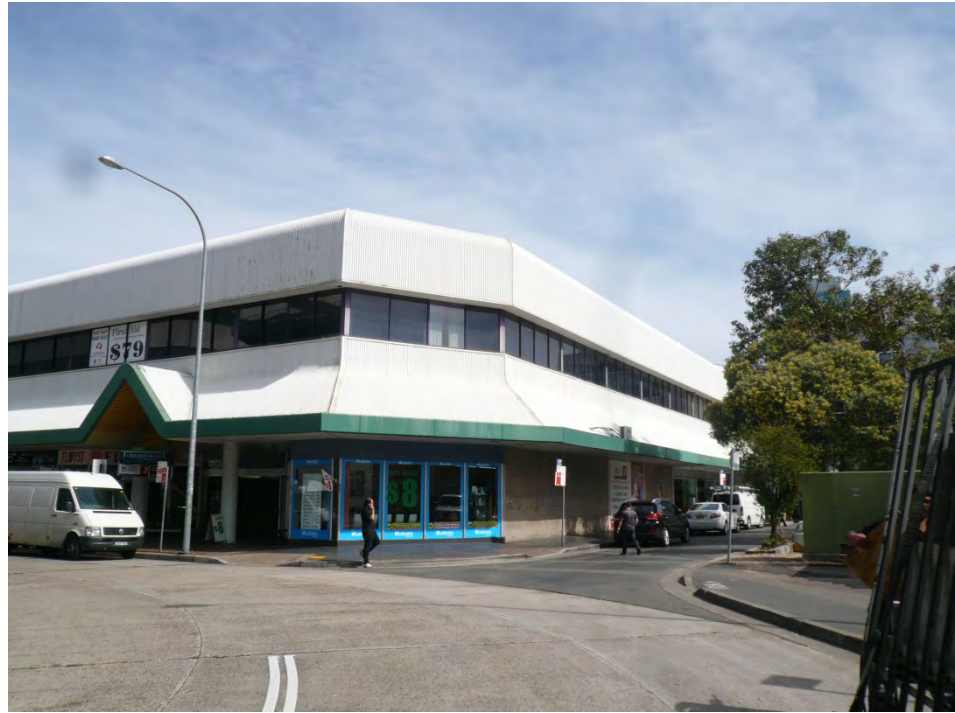
Figure 7 – View of site on the corner of Horwood Place and Houison Place
