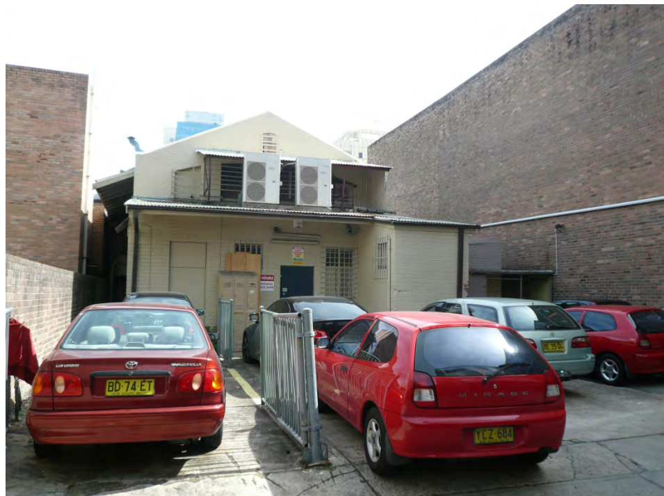
Figure 8 – Rear view of site (No. 220 Church Street)
